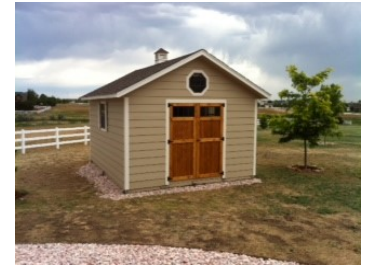
Hardi-Lap siding (concrete)
